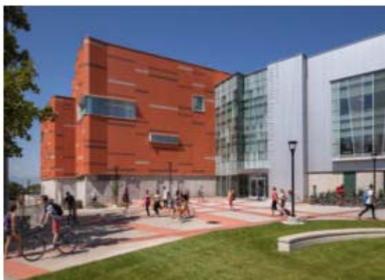
North View of South Entrance of ESLC
